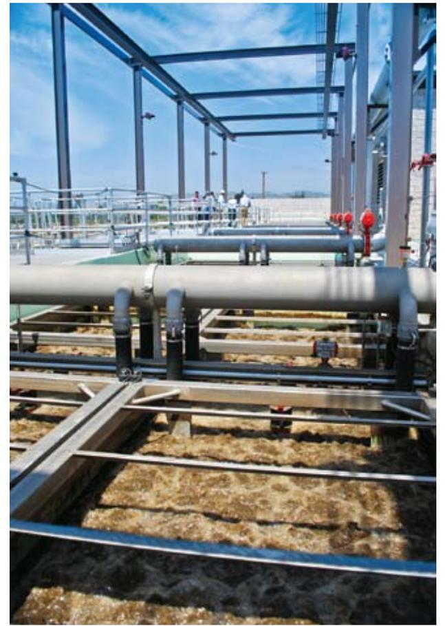
Most of the wastewater treatment takes place in underground MBR tanks.
